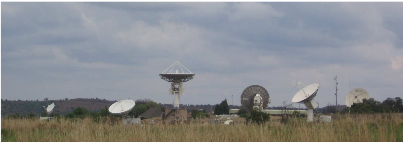
Figure 44: The CSIR Satellite Applications Center at Hartebeeshoek near Johannesburg. Special antennae track satellites as they pass overhead and download images using radio waves.
